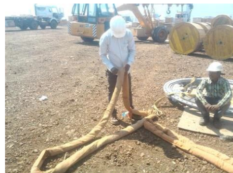
Inspection of Lifting Tools & Equipments at Nipaniya
